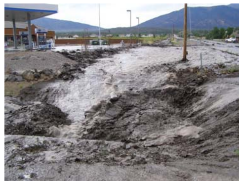
Flooding downstream of the Schultz fire
