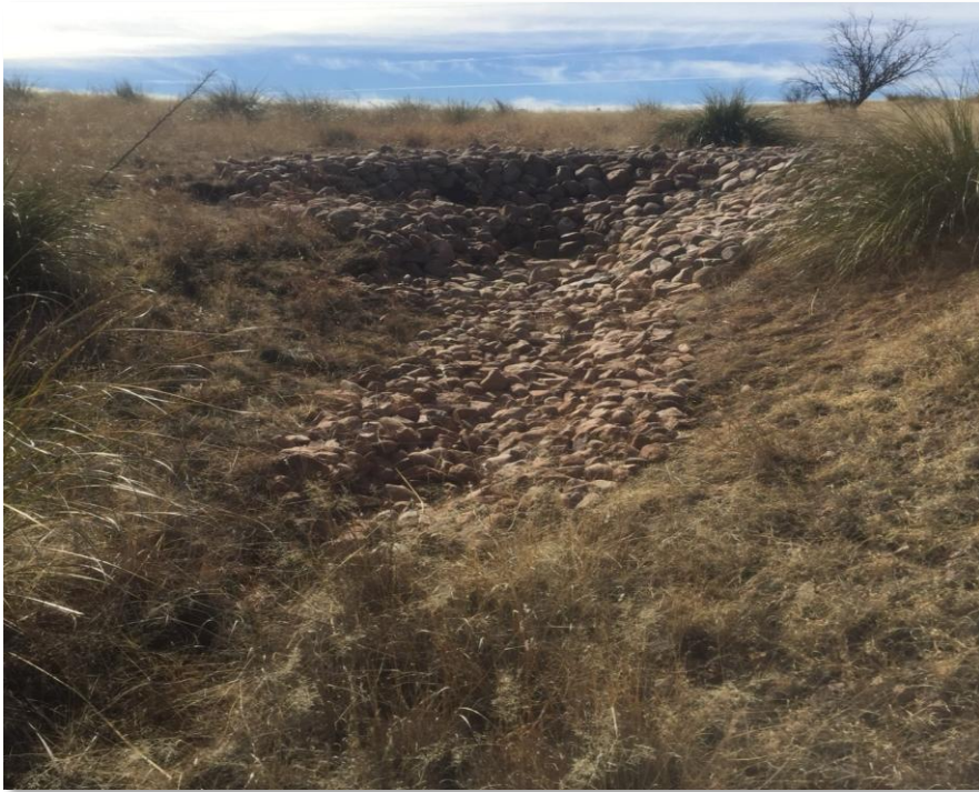
Zuni bowl arresting erosion of a head cut in an Arizona grassland.
