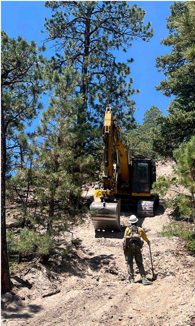
An excavator is used to rehabilitate firelines and roads following the Indios Fire. Credit/ Marija Osipchuk/BLM
